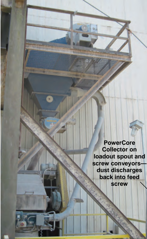
Volumetric Feeder & Eductor Transfer System Delivering Magic Powder To Treat Baghouse Containing Hazardous Dusts
